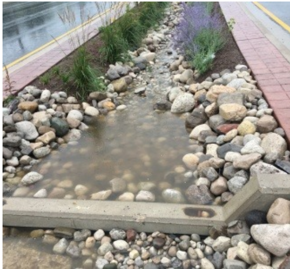
Figure 8. Check Dam Inspiration
